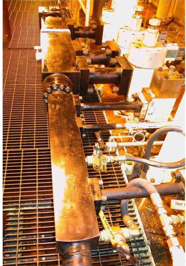
ANSI 1500# Multi-Port Block Header for OSB Plant
